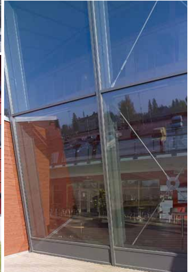
Clean transitions in a complex location with specially designed cover plates between the large slanted and curved glazed surfaces.
