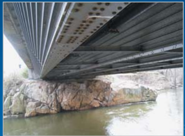
Virginia Route 36 Bridge over the Appomattox River in Petersburg, VA
