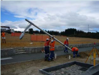
Placing light weight aluminium columns
