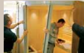
The aluminium profiles round the opening are put in position.
