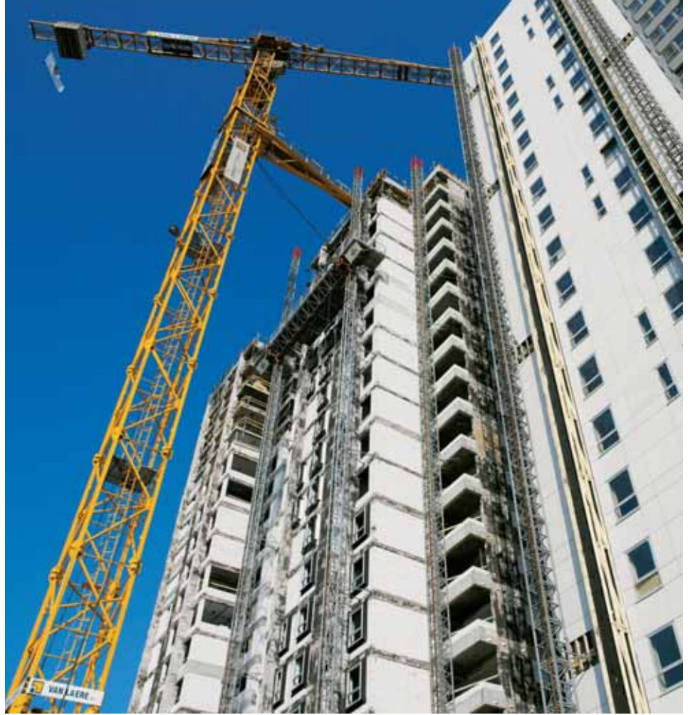
New window frames give Silvertop Towers better soundproofing and thermal insulation.
