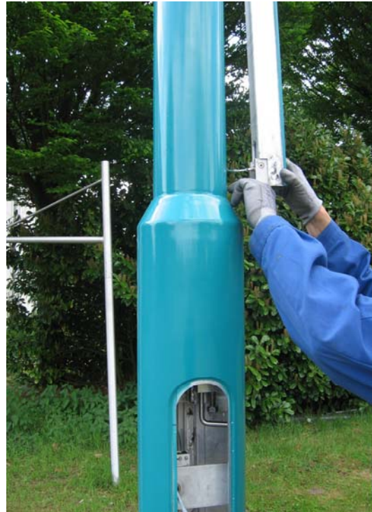
Pic. 14 At the end, note that the ribbon isn't twisted and goes in the column without any knots.
