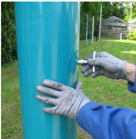
Pic.01 Unscrew the 2 special bolts from the door.
