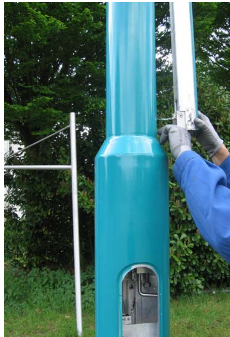
Pic.08 Bring the arm just past the dead point with your hand.
