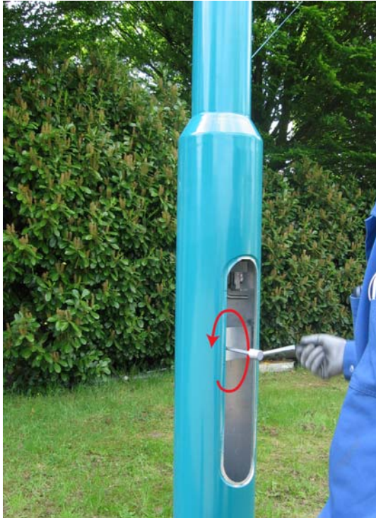
Pic.09 Tilt the column by turning the winch to the left.
