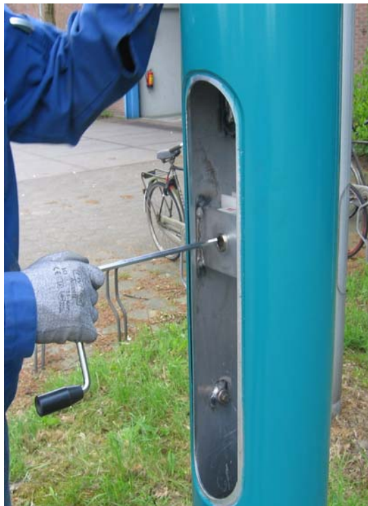
Pic. 15 Take the lifting handle out of the winch.
