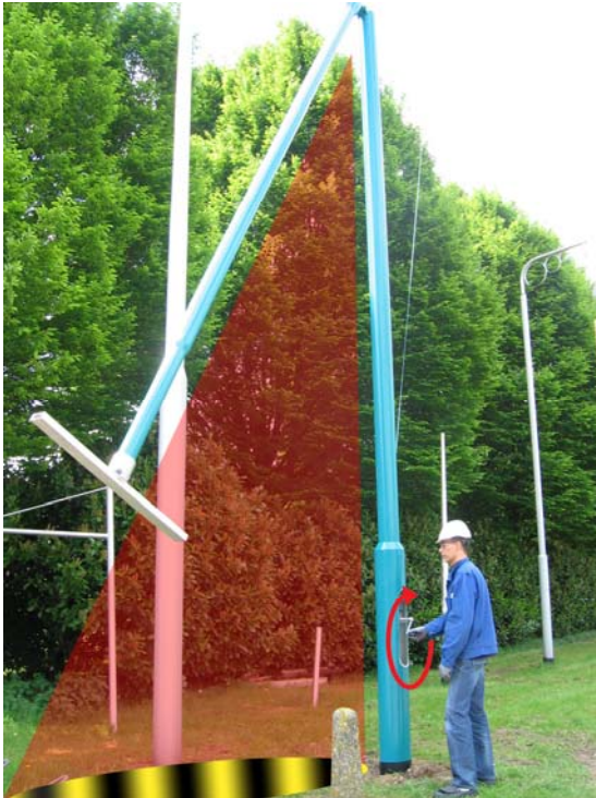
Pic. 13 Turn the winch Clockwise to see the column right. Note: Don't stand between the column and arm during operation.
