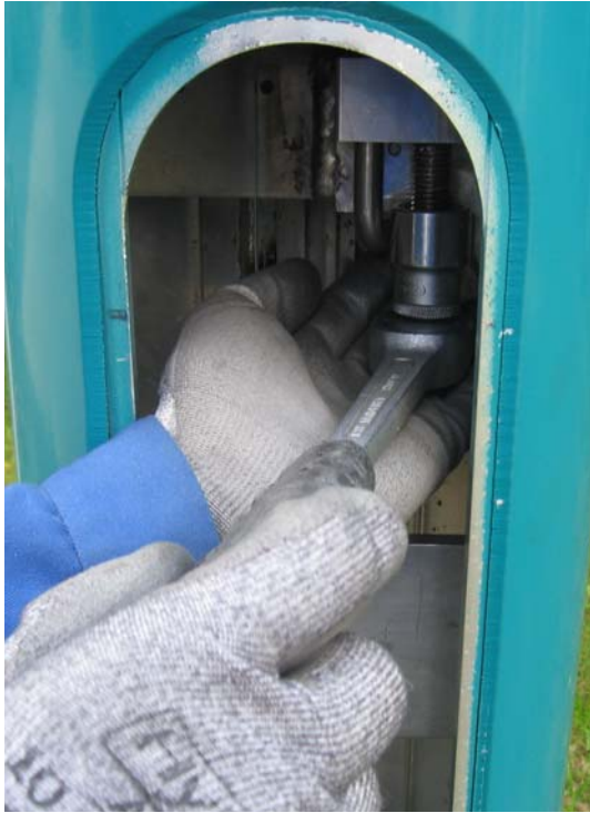
Pic. 17 Then tighten the locking bolt with the tool. (dimension across flats-24 mm)
