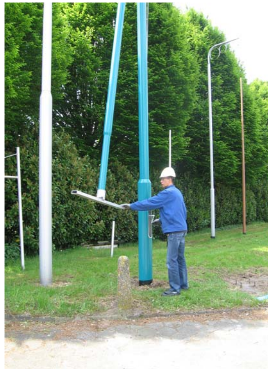
Pic.12 Keep turning until the column is tilted to the buffer. Make sure that the column is lowered slowly.
