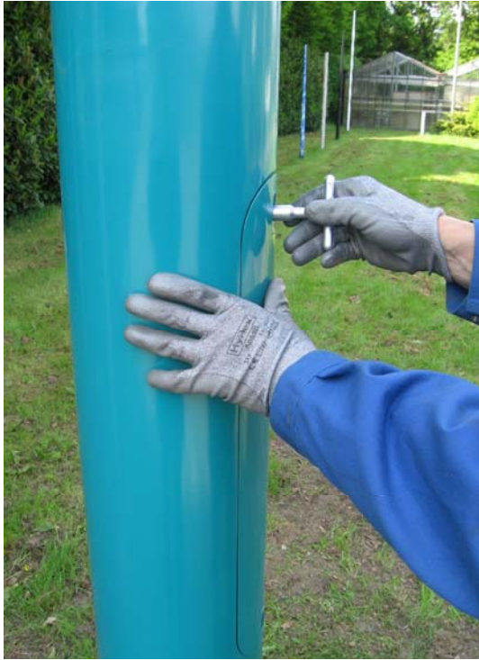
Pic.21 Tighten the 2 special bolts to the door.
