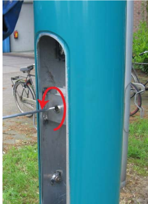
Pic.06 Install the lifting handle into the winch.
